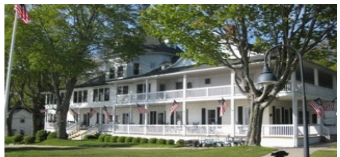
Now known as the Community Center, the Epworth Hotel was built in 1894.
